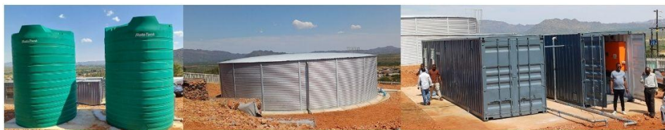
Bodutlolo Water Supply Project at Ga-Mathabatha
